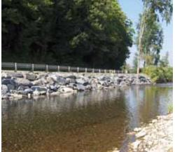
A road is located in close proximity to the river. Along with negative impacts of failed riprap along the banks, it also becomes expensive to continue to maintain riprap to protect infrastructure that is placed in the river's meander path.
