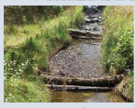
Cascade (above) with excavated floodplain at lower end of project site to arrest the headcut and restore floodplain function. At right, re-established riparian vegetation.
