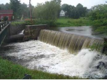
This is a photograph of a small impoundment at Cilley Hill in the Browns River watershed, where the flow is slowed above it and the power of the release deepens the channel below it.
