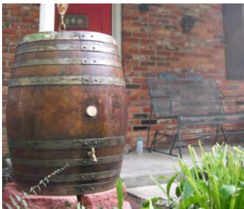
RAIN BARREL. Collects and stores stormwater from guttered roof downspouts. Water can be used later for activities such as car washing or irrigation.
